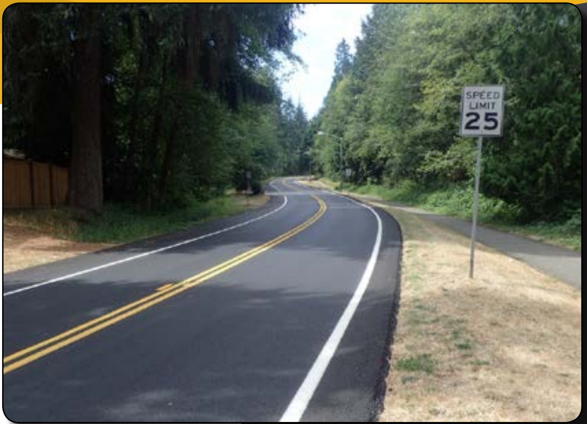
Completed Overlay - Somerset Hill Road
