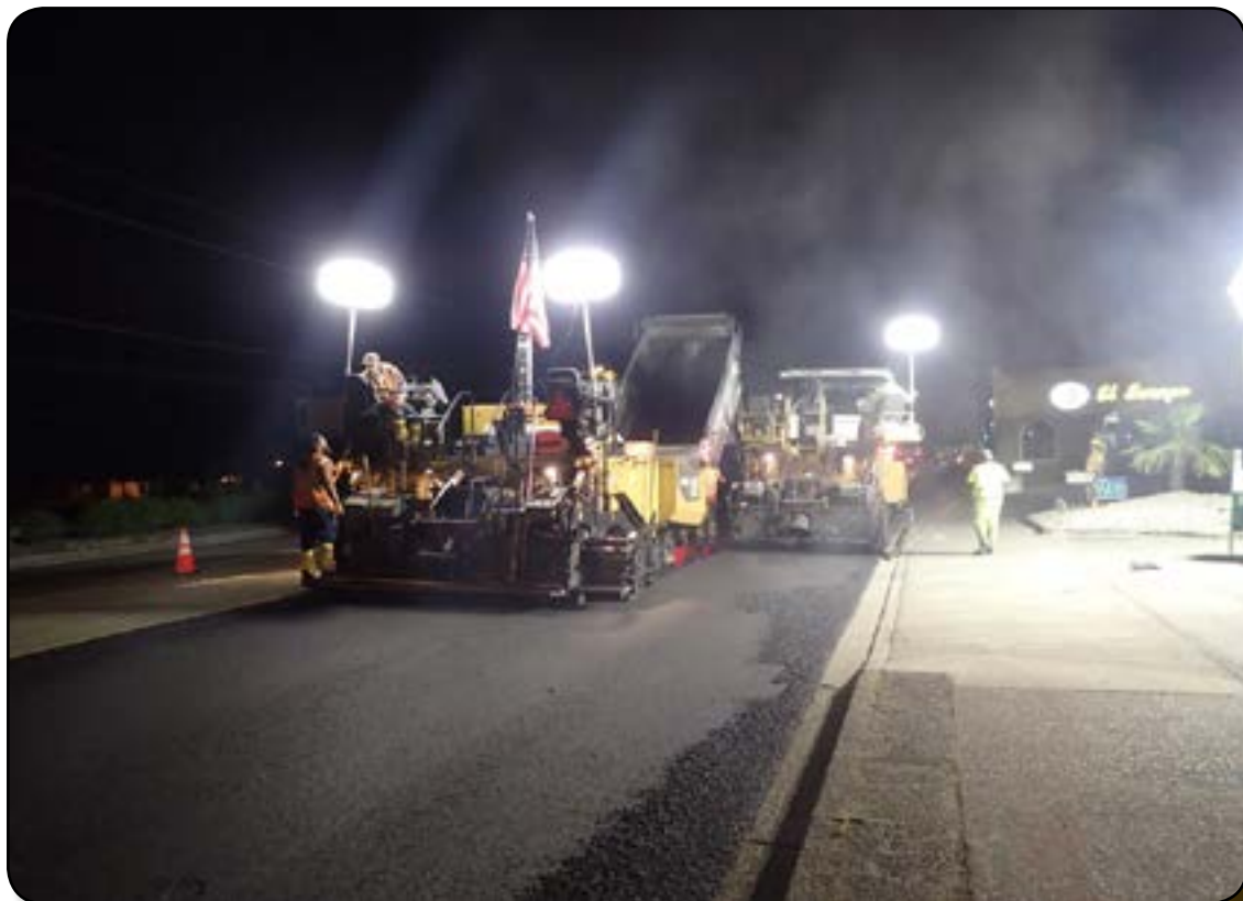
Capitol Blvd – Night Paving
