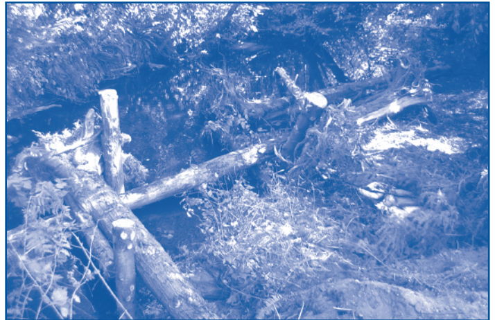
▲ Newly installed wood structure at Black Lake Ditch.
