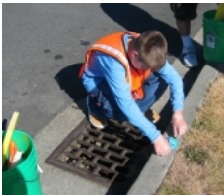
Applying a storm drain marker in Streamland Estates.
