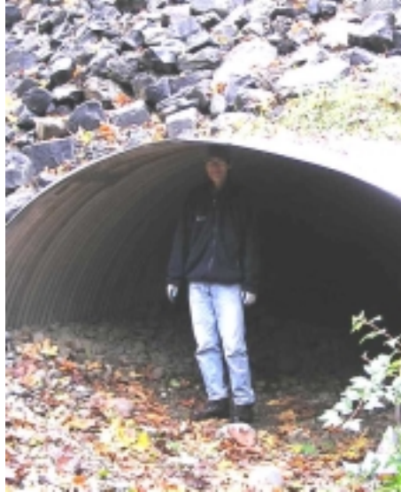
Terence checks out the Perkins Creek culvert.
