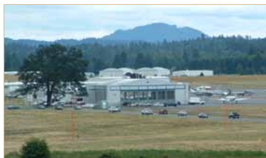
Old Olympia Airport Hanger/Terminal at Olympia Regional Airport
