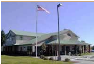
Tumwater Fire Department headquarters
