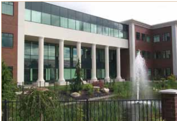
Point Plaza courtyard
